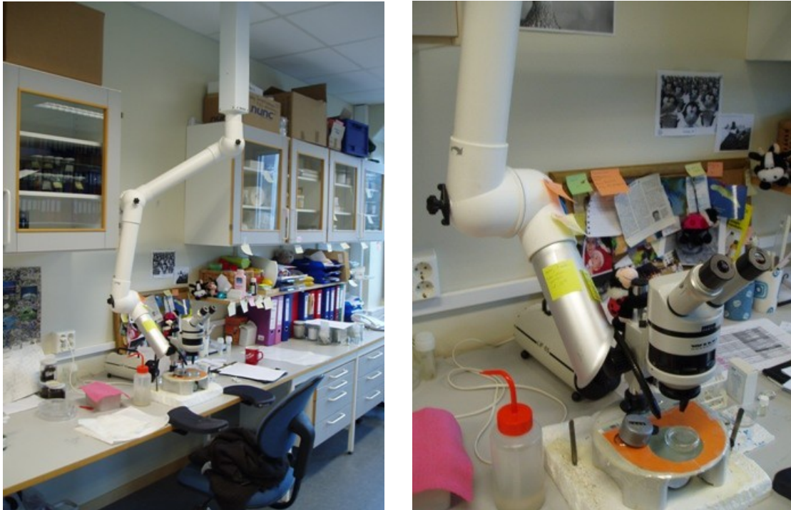
Figure 6. This point-ventilation outlets can be an alternative for short period of time. We use this for ethanol-samples. Visit the web at the following address to see some different solutions. http://www.alsident.com/
