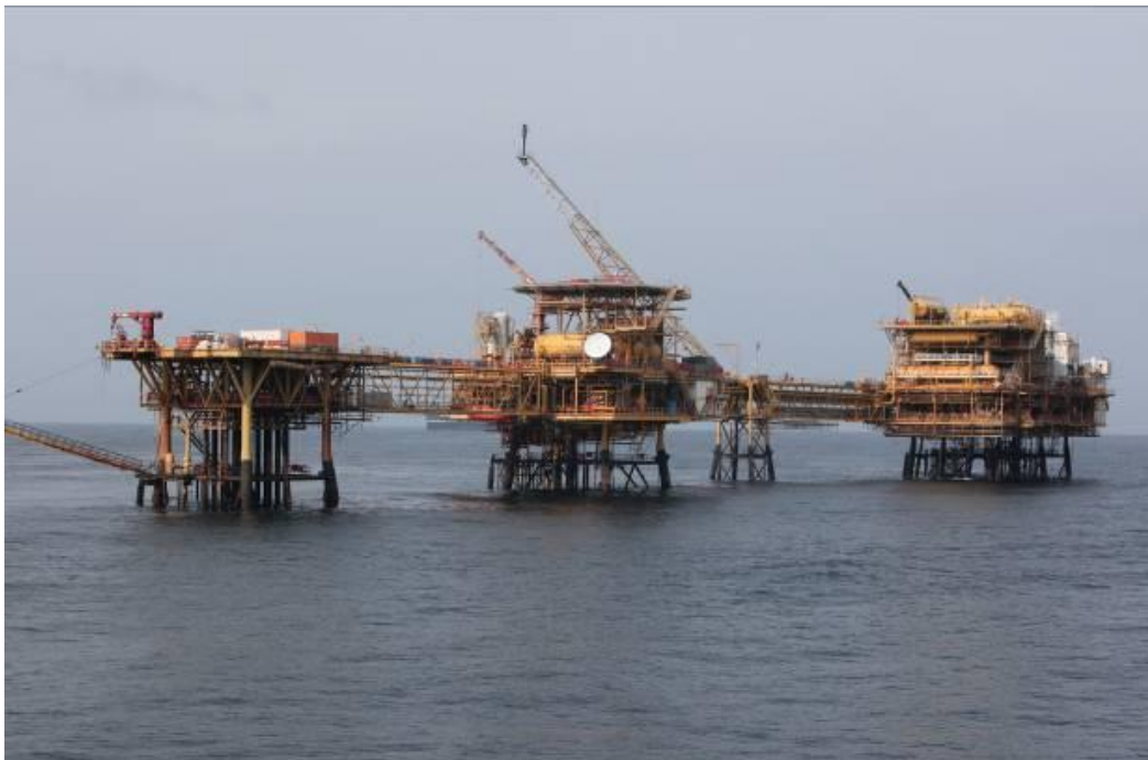
Picture 7.1. The Palanca platform.
