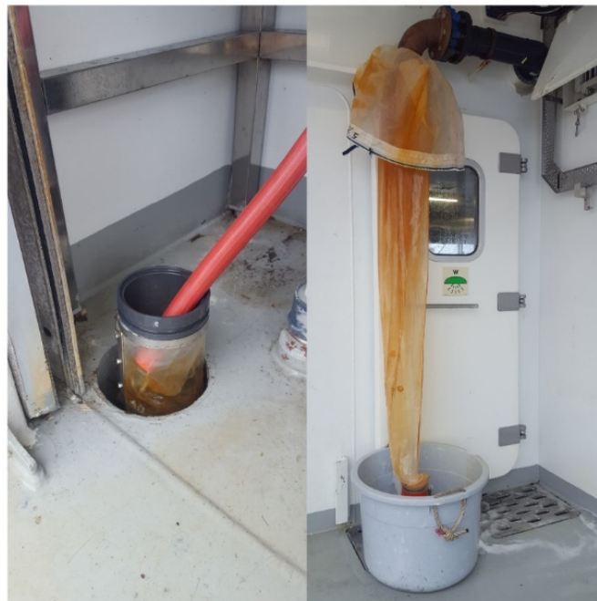
Figure 5. "Small water pump" and "Big water pump – CUVES". Image credits: Alina Rey
